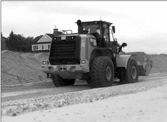
The front end loader helped move around the 5,000 cubic yards of new sand to reinforce the Spit in anticipation of winter storms
