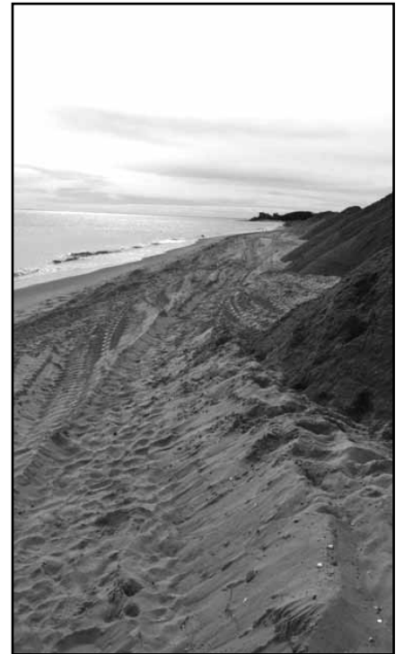
The Barnstable County dredge arrived in mid-April and dumped 9,000 cubic yards from the outer channel onto the Spit.
